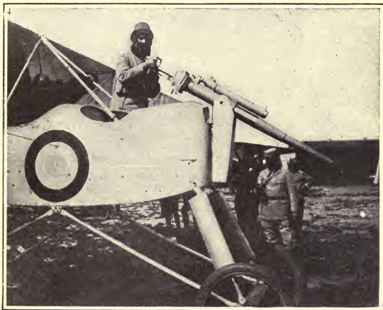
FRENCH AVION-CANON MOUNTING ONE 1½ IN. Q. F. GUN
